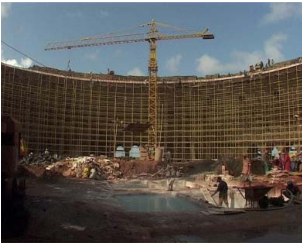
Construction of the dome of the Global Pagoda, as of June 2005
